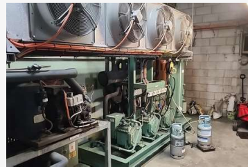
Essential maintenance of rack system
